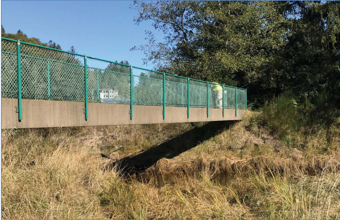
Figure 6-1. Aboveground crossing of transmission main
