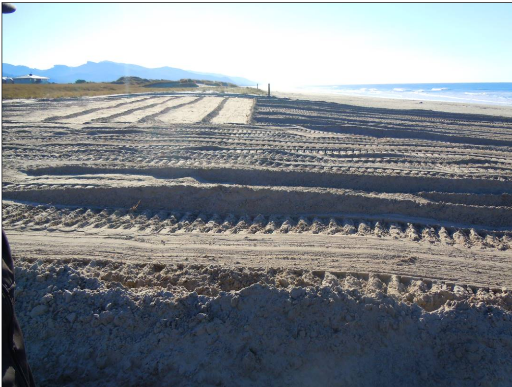
Figure 30: Design Foredune Configuration calls for the 25 ft NGVD bench (left). Sand ramp slopes down to the upper beach and becomes a grassy foredune unintentionally.
