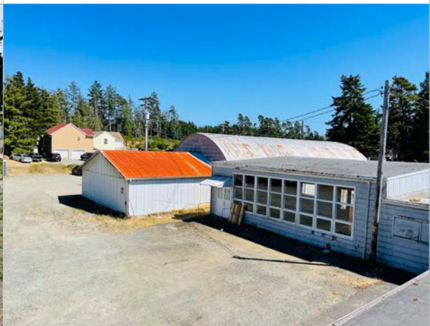
Exterior of Buildings 2, 3 and 4: South Side
