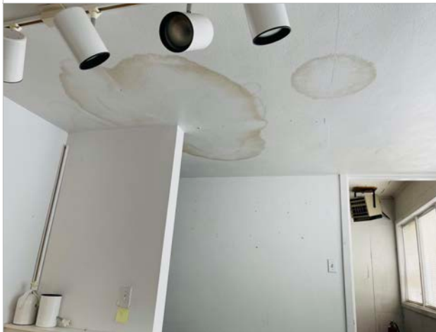
Example of Staining: Staining observed on ceiling
