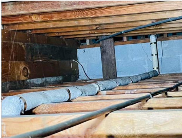
Attic Above Areas 3 and 6: Asbestos-containing pipe insulation and fittings
