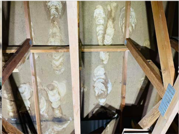
Example of Staining/Mold Growth: Staining and mold growth observed on ceiling
