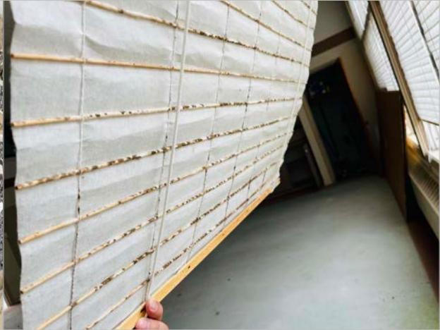
Example of Mold Growth: Mold growth observed on window shades
