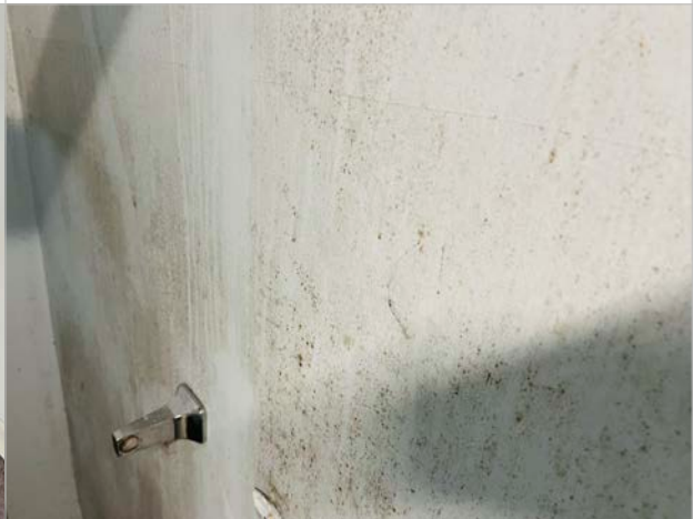
Example of Mold Growth: Mold growth observed on interior wall
