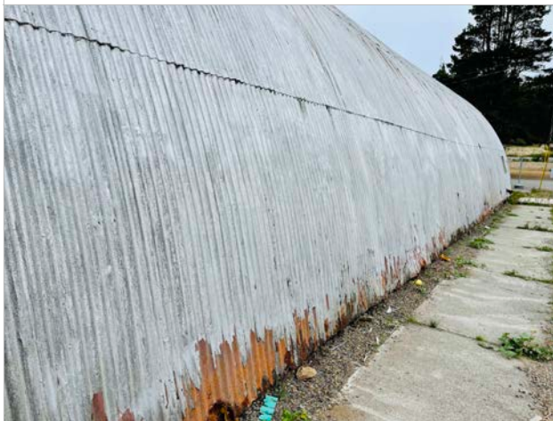
Exterior of Building 3: Asbestos-containing silver coating
