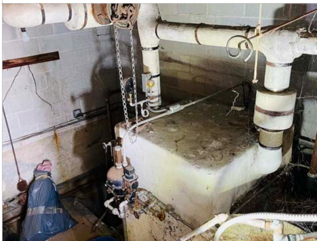
Boiler Room: Asbestos-containing boiler insulation, pipe insulation and fitting insulation
