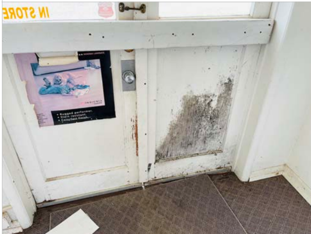
Example of Mold Growth: Mold growth observed on interior of door
