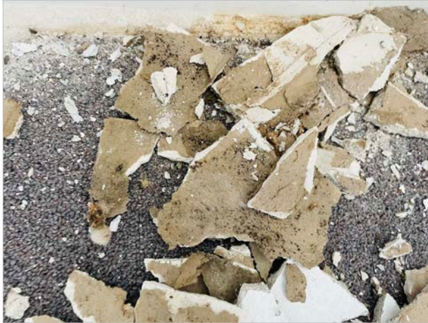
Example of Mold Growth: Mold growth observed on wallboard, on the interior of the wall cavity
