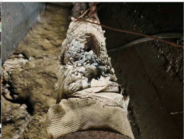
Boiler Room: Example of damaged asbestos-containing pipe insulation
