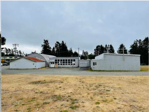
Exterior of the Site: South Side
