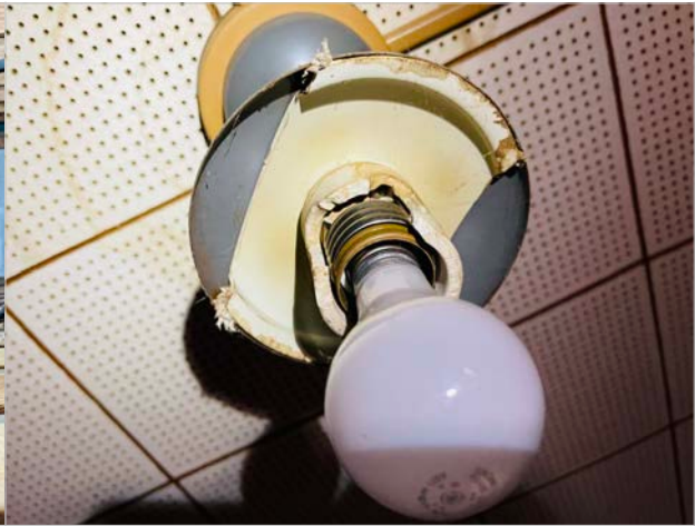
Example of Light Fixture: Asbestos-containing insulation
