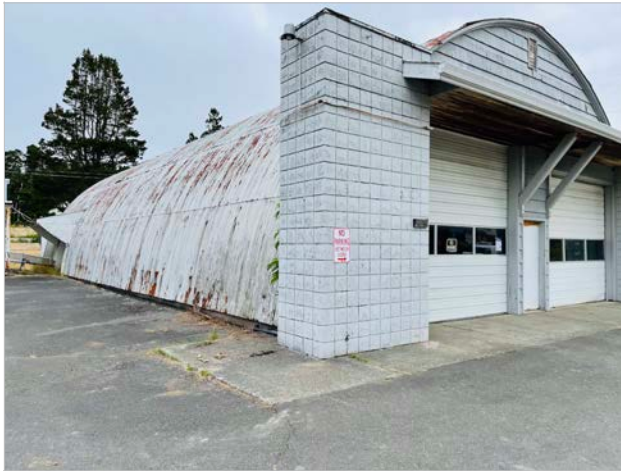
Exterior of Building 3: SW Side
