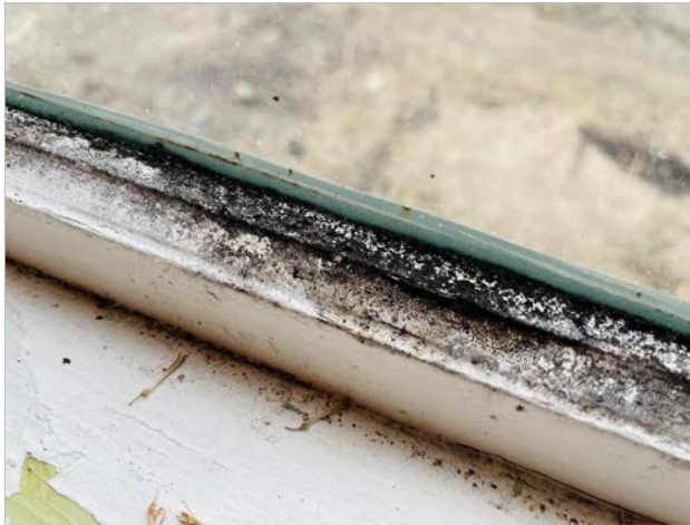
Example of Mold Growth: Mold growth observed on window
