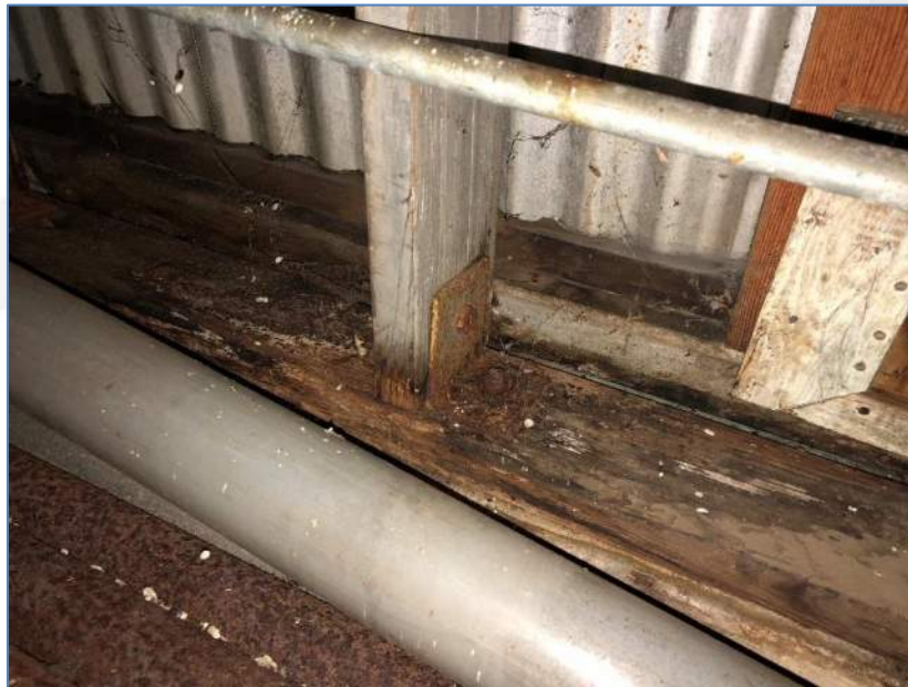
Figure 8: Rusted Glulam Arch to Foundation Connection
