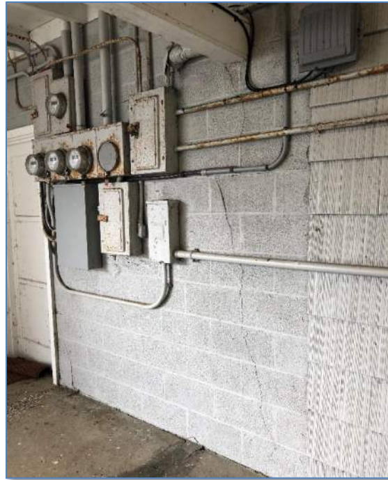
Figure 6: Cracked CMU Wall and Outdated Electrical
