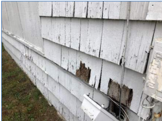
Figure 1: Deteriorated Siding
