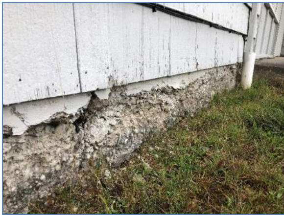
Figure 3: Foundation Deterioration
