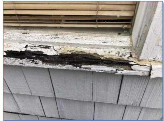
Figure 2: Deteriorated Window Sill
