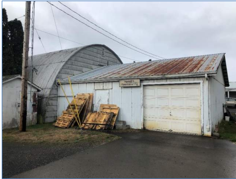
Figure 9: Storage Structure Deterioration
