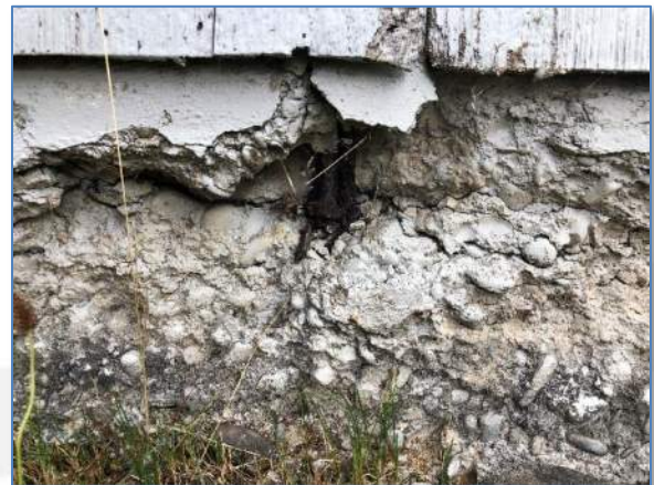
Figure 4: Exposed Anchor Bolts
