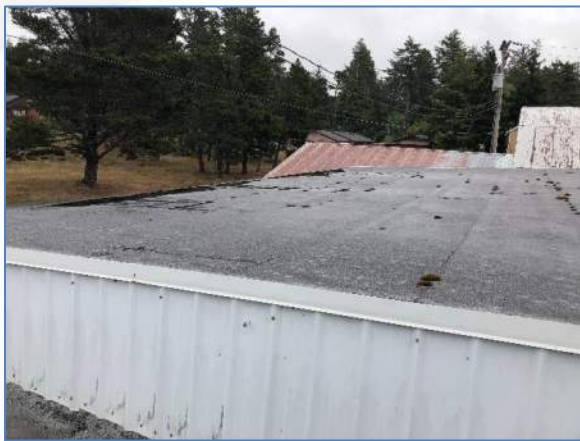
Figure 5: Roof Ponding and Moss Buildup
