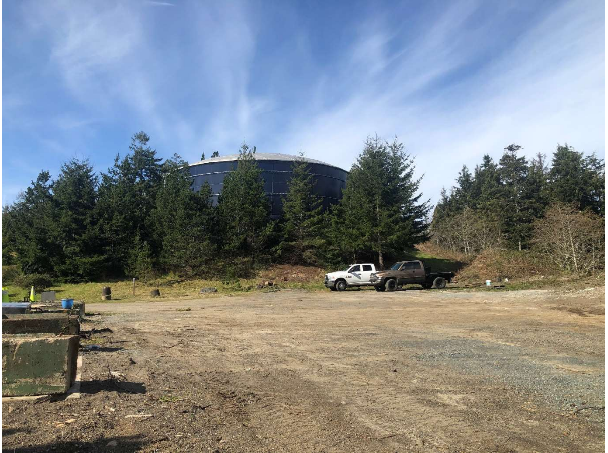
Exhibit 3-2: Gravel lot east of Reservoir No. 3. Lot is built on approximately 20-feet of uncompacted, undocumented fill.
