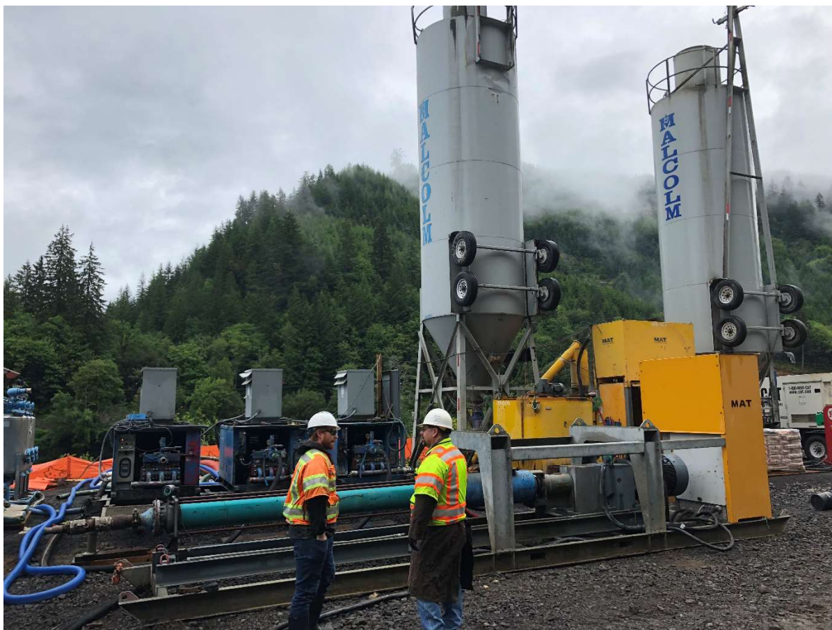
Exhibit 7-2: Photo of deep soil mixing plant at OR 38 Scottsburg Bridge.
