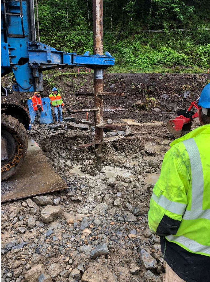
Exhibit 7-1: Photo of deep soil mixing paddles at OR 38 Scottsburg Bridge.
