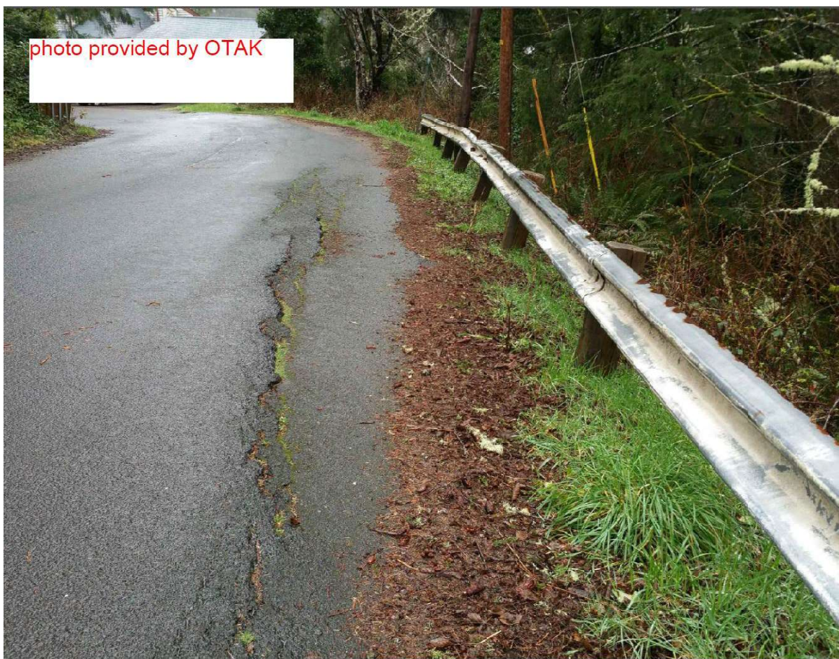
Exhibit 3-7: 2017 Surface cracking and deformation along Epoh Avenue.
