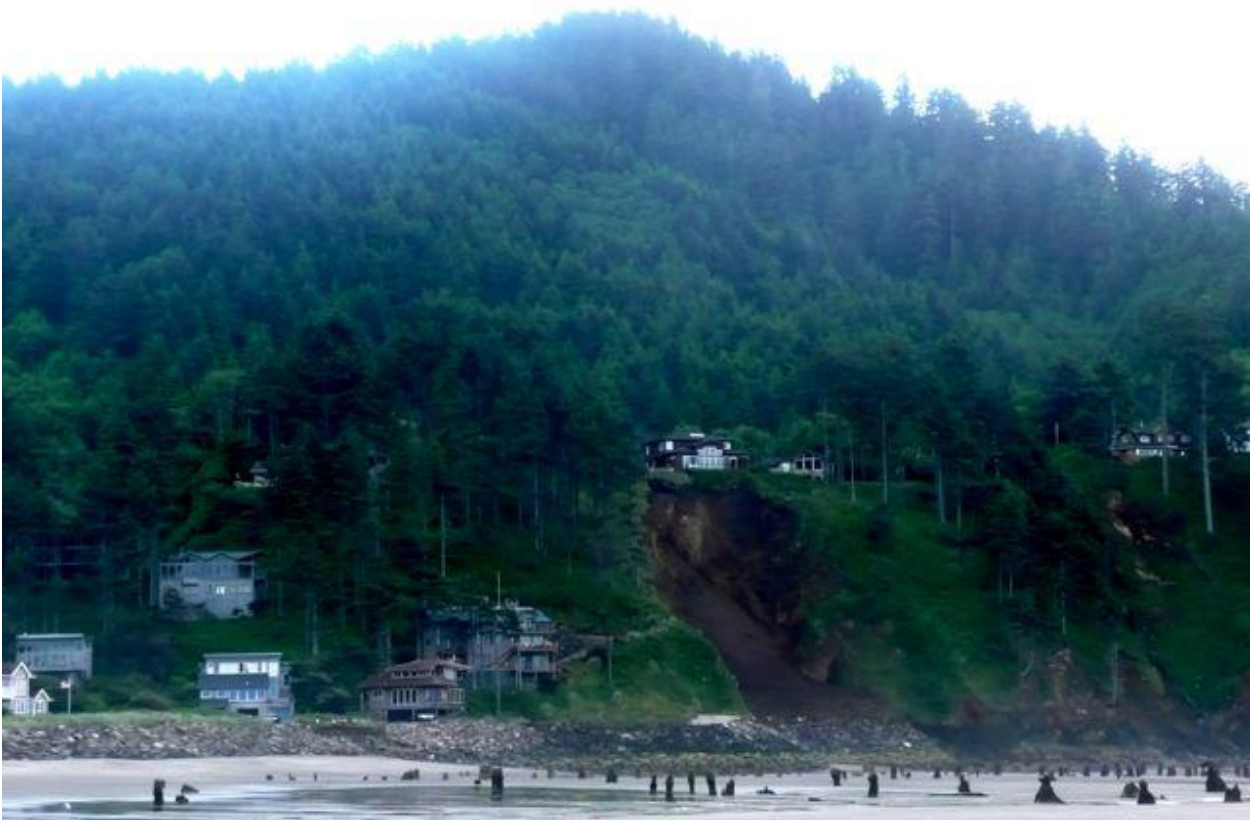
Figure 63. Landslide in Tillamook County
