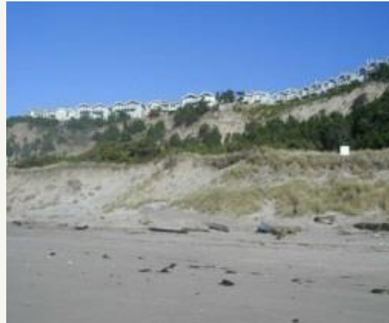
Figure 31. Erosion at “The Capes” Condominiums, Oceanside, Oregon
