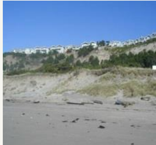
Figure 31. Erosion at “The Capes” Condominiums, Oceanside, Oregon
