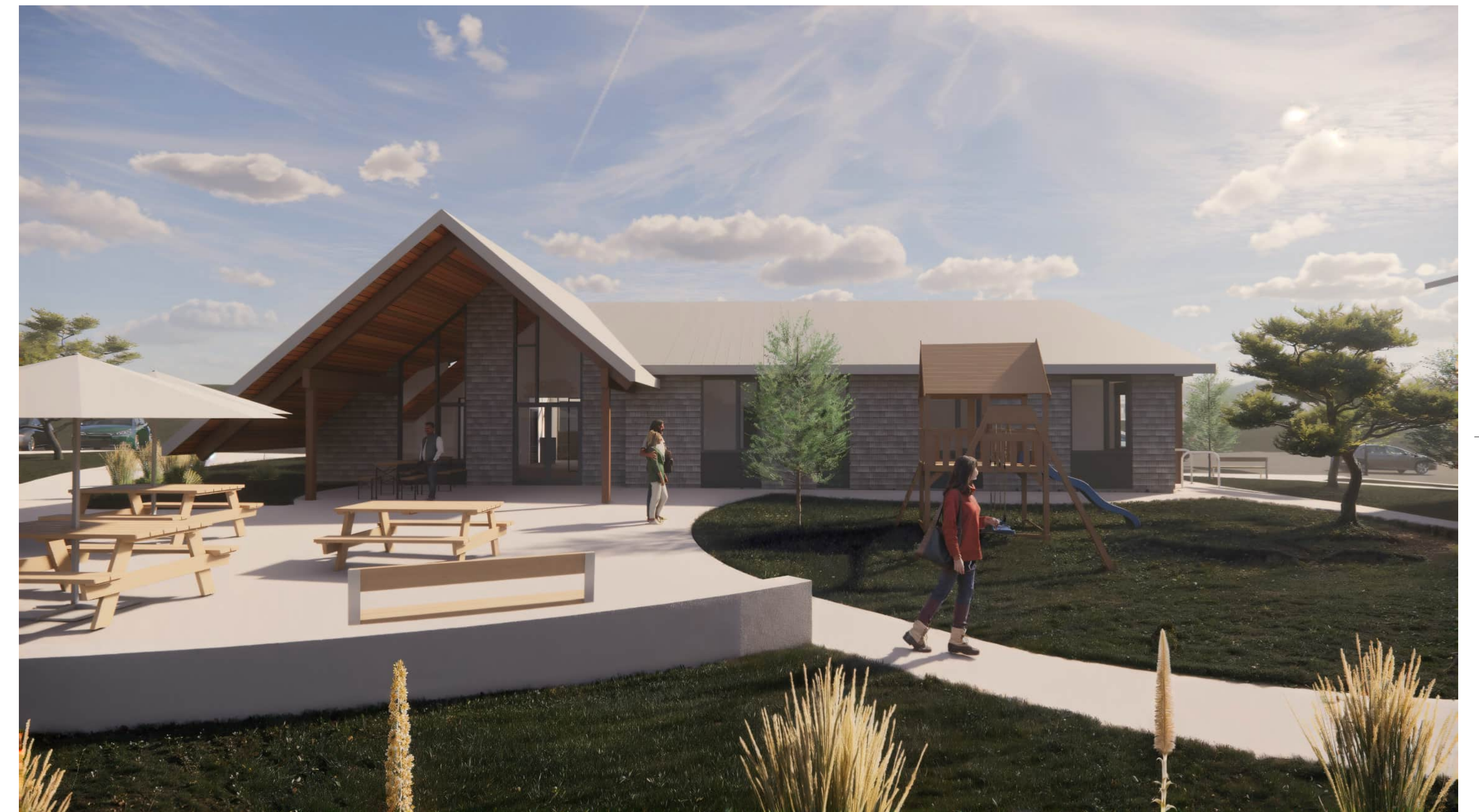
ABOVE: VIEW OF WEST FACADE OF CLUBHOUSE
