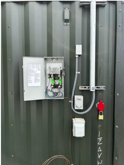
Exterior 100-amp service disconnect Interior Sub panel on Secondary container
