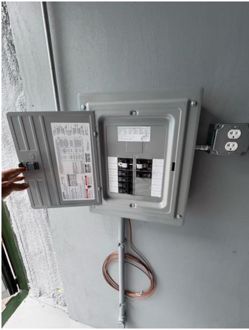
Exterior 100-amp service disconnect Interior Sub panel on Secondary container
